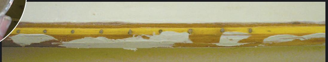
'We stuck wedges into where the wood was splitting, forcing the crack open to allow the air to circulate and allow any moisture that had got inside to get out.
